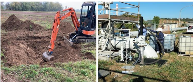
FIGURE 1: Excavation (left) and Leakage Tests (right)
